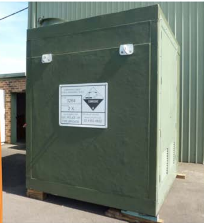
CDU2.5 Chemical dosing unit
