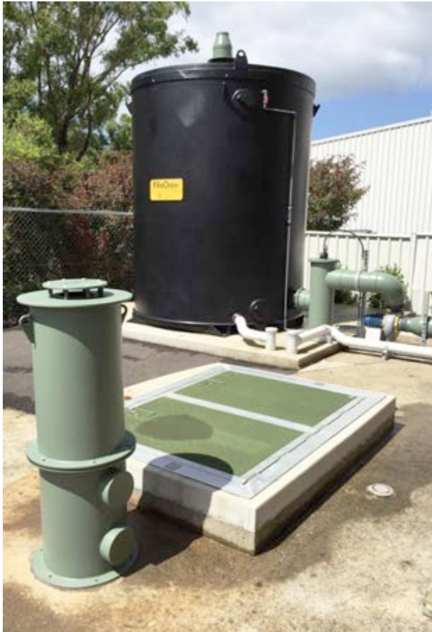
FiltaOdor™ F0300 with a FiltaVent™ two-way passive filter in foreground installed for Coffs City Council WWPS (Waste Water Pump Station)
