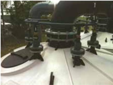
**Figure 1. View of RICF roof showing wash system.**
