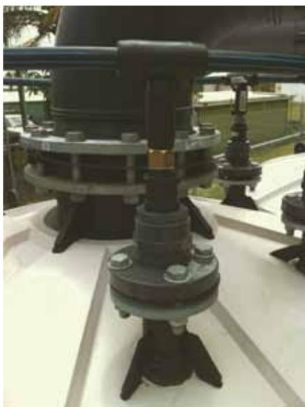
Figure 5. Washing nozzle assembly.
